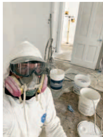
Paul gets ready to paint
