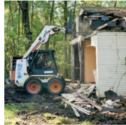
Jim Mayer knocking down the Fox Den.
