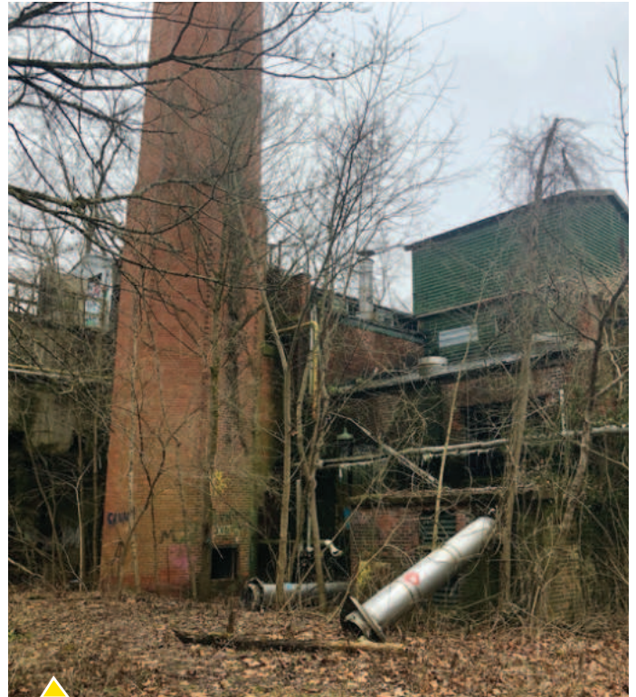
The Antioch College coal-fired power plant.
