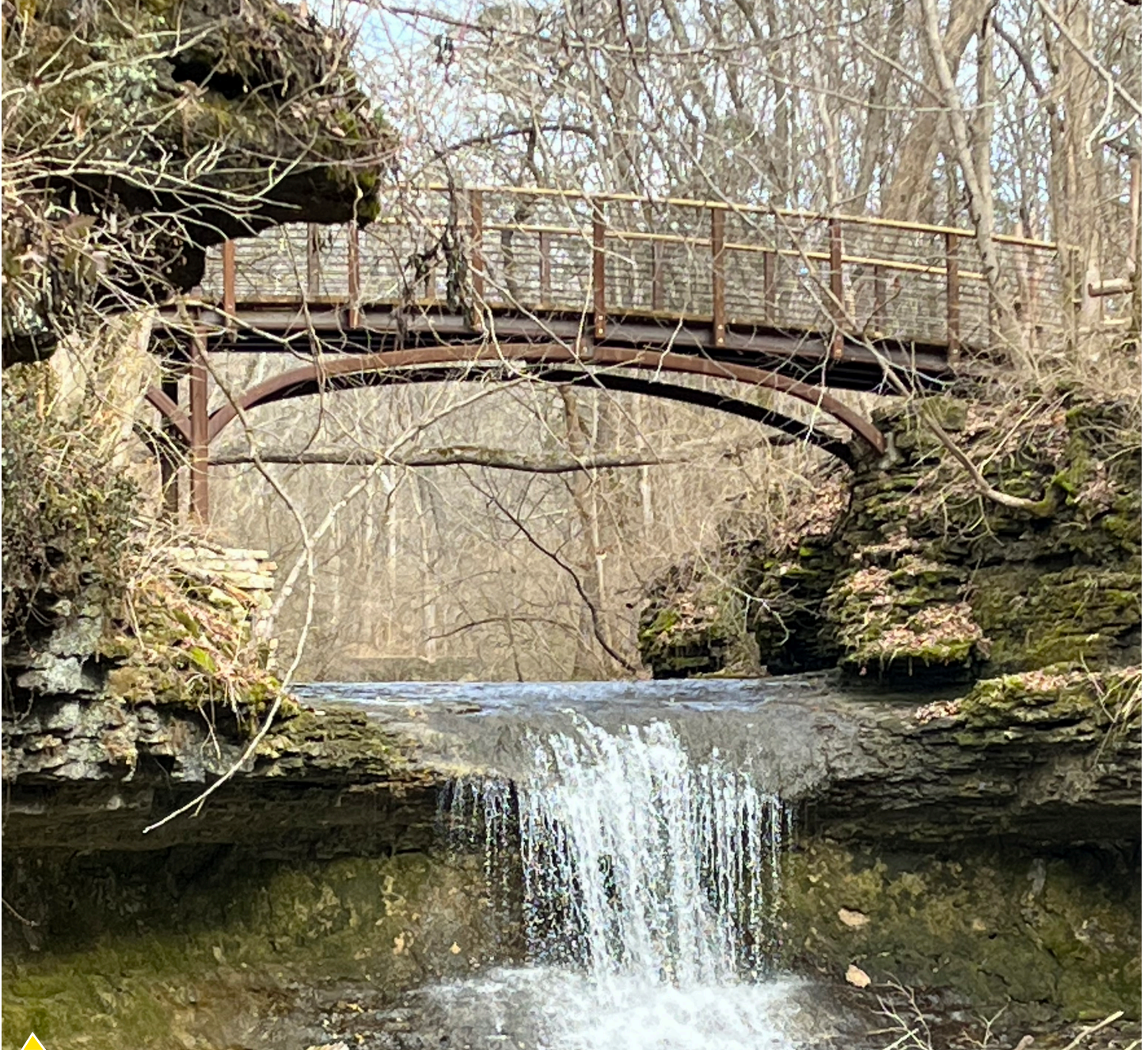
The beautiful new bridge over the Birch Creek Cascades
