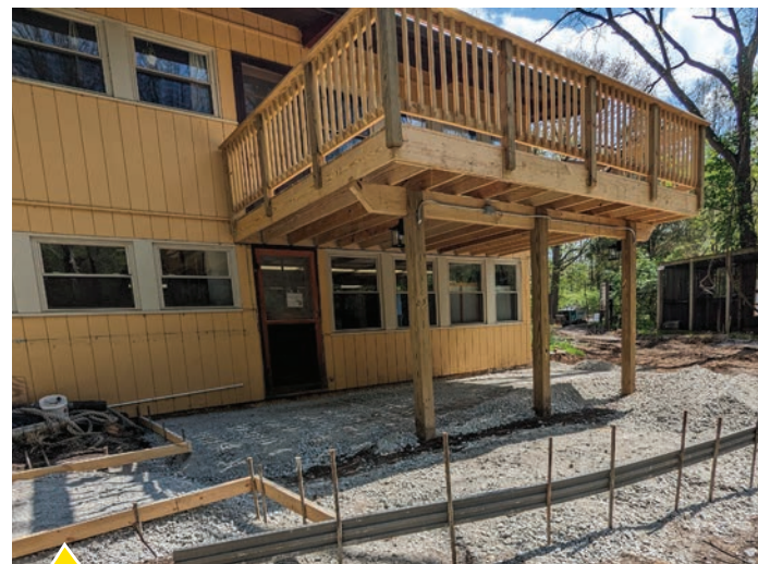
The new ADA compliant sidewalk takes shape around the raptor enclosures.
